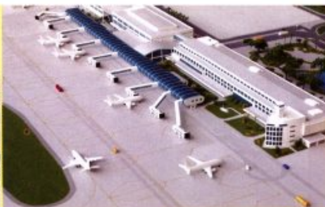
Reforma e ampliação do Terminal de Passageiros, do sistema de pistas e pátios e obras complementares (maquete) | Restructuring and expansion of the passenger terminal, the runway and patio system, complementary works (model).
