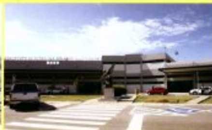
Reforma e ampliação do Terminal de Passageiros, Administração e Torre de Controle | Refurbishment and expansion of the passenger terminal, administration building and Control Tower
